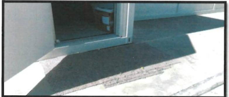
10. Se identifica varios desniveles defectos en el piso de vinil. / The joined containers (HDU/ICU/ DINNING ROOM/ BATHROOMS AND DOCTOR ROOMS) present several defects due to difference in levels between them.
