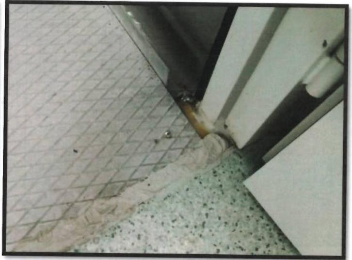
8. Rampa en las puertas de emergencia/ Due to the level difference, ramps in Emergency Doors are needed.
